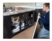
Remove the spa panel for access to spa components. Reverse these steps to reattach the spa access panel.
